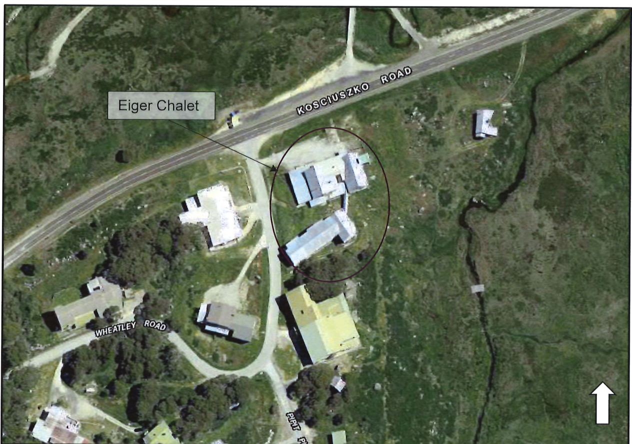
Figure 1: Eiger Chalet (Source: SIX Maps 2019)
