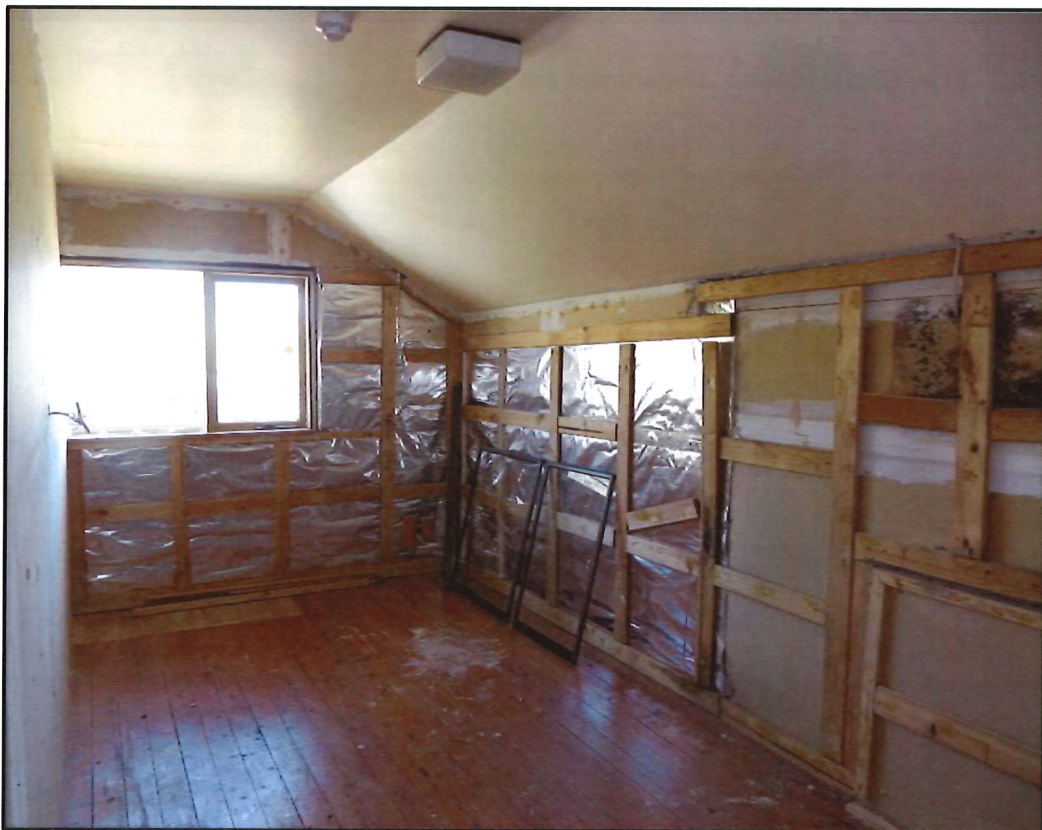
Figure 3: Eiger Chalet guest apartment (Source: site inspection photo 2019)
